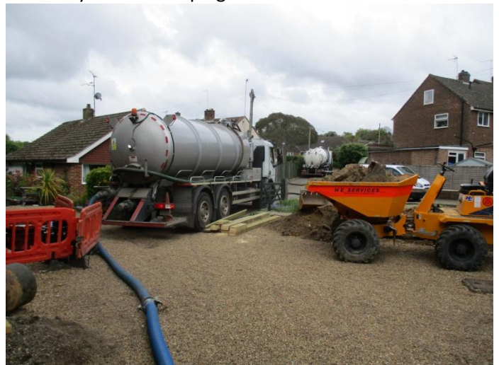
Standby tankers keeping excavations clear
